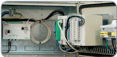
I/O units are mounted in the apparatus compartment. Connection to central unit is made with a modular cable
